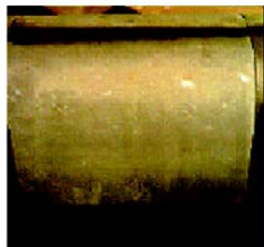
Lower RCC Panel Surface
